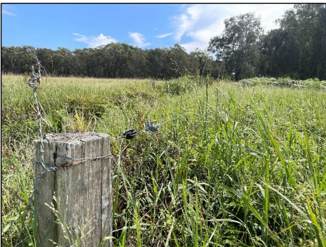
Plate 5: Agricultural improvements within the Project Area include livestock gates and fencing in disrepair.
